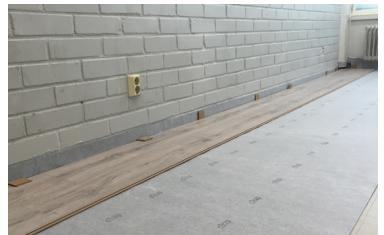
**N.B!** It is the fluffy side that must lie against the surface from which the emissions are spreading. You should be able to see the text "cTrap" when the cloth is in place. For best results the cloth should be kept dry even after installation.
