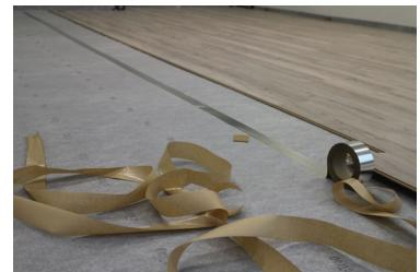
**When attaching on a floor**, flooring that does not require to be glued may be laid directly on the cTrap cloth. In other cases, the flooring is glued to an underlay which is laid on the cloth.
